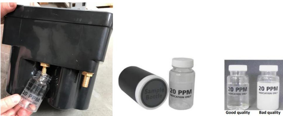
Figure 19. Oil- water separator with sample bottle
